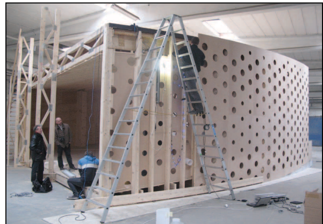
Figure 5: full-scale, wood model of a section of the facade
